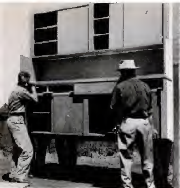
Prebuilt kitchen cabinet wall made of hardwoods is moved into a new May home
